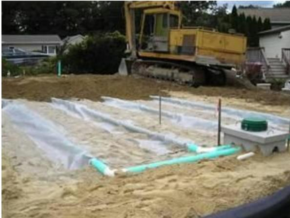
The leaching area which the water is pumped to can be configured in several ways. Being elevated, the engineer must be aware of the soil composition so any chance of erosion, contamination or worse yet flow back to the property can be avoided. In a location with ample space, the leaching area can be placed far enough away from the home to eliminate the chance of this. In locations where this is not possible, the
