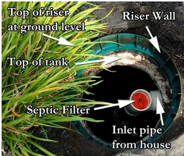
This graphic shows a riser which was added to the septic system. It shows how the inspector needs only to remove the riser cover to gain access to the septic tank. You can see in this image how the inspector has direct access to the filter and septic tank to perform his inspection and maintenance of the tank.
