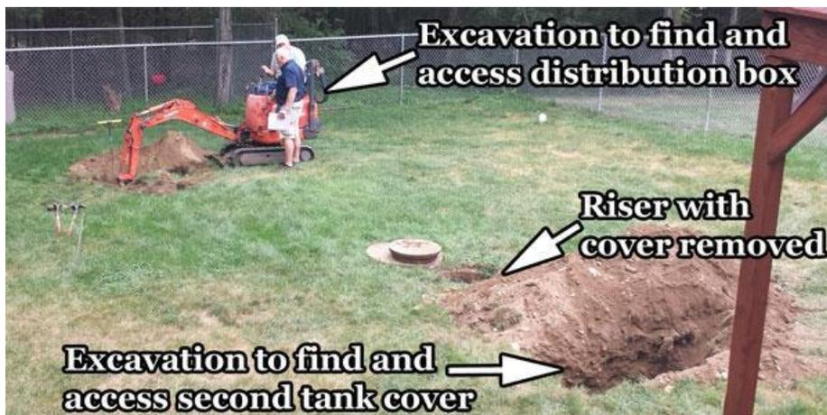
This is a picture of a septic system with only one riser. As you can see, the inspectors required an excavator to dig down to the septic tank and distribution box access covers. This
